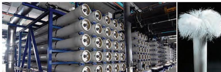
but solids can't. Thus passing Water through the membrane is expected to clean the Water up to some extent. There are many technologies as a subset of membrane technology like Reverse Osmosis (RO) technology, pressurized filtering through the membrane, high-pressure filter-
